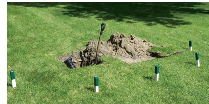
Mark off repair areas.
